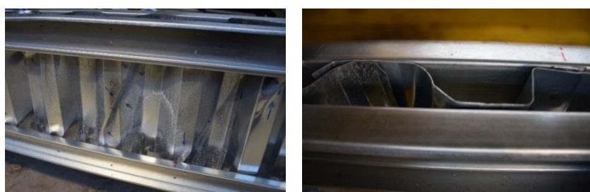
Figure 13: Distortion of the web corrugation of the CWB SW-1 beam.
