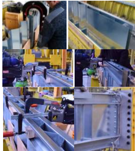
Fig. 7. Stages of beam built-up.
