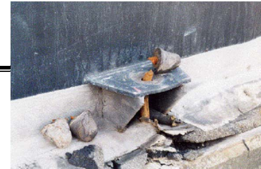
Cut off of anchor bolt
