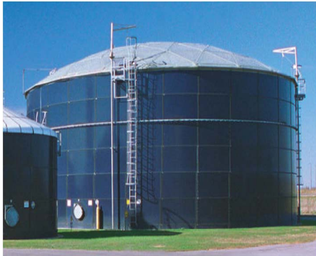
Storage tank, dome roof
