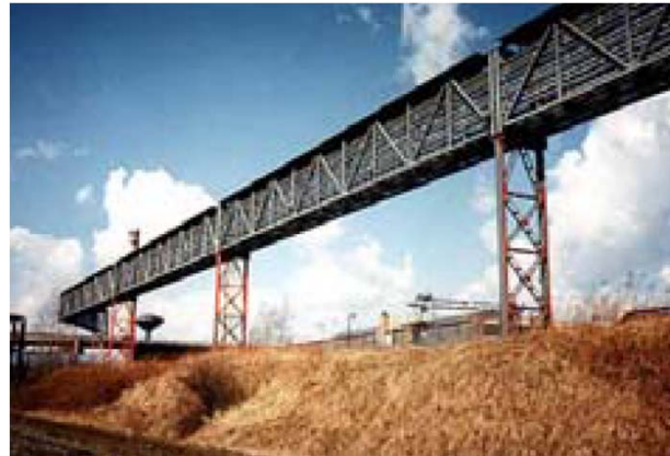
Pipeline bridge - general view
