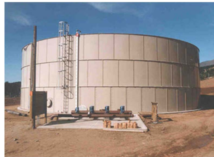
Irrigation Water Storage Tank
