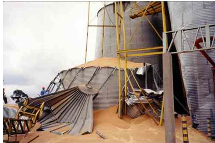
Failure of a grain silo
