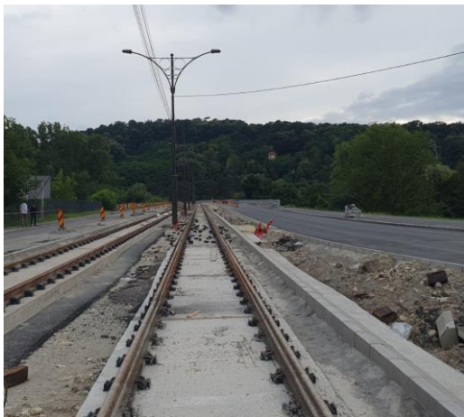
Figure 2. The current situation of the tramway, the Intim bridge area
