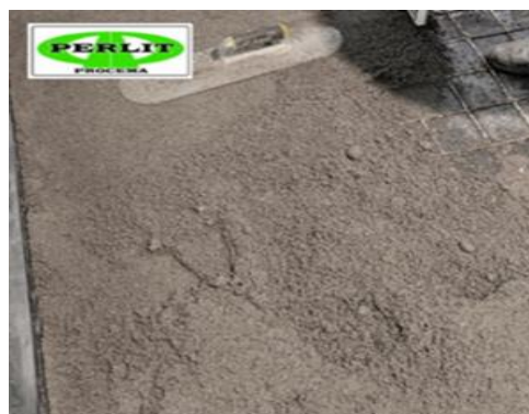
Figure 4. Stabilized perlite used for thermal insulation of floors above basements and as a trench support layer. [1]
