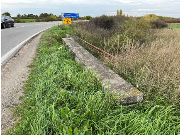
Figure 1 Existing footbridge, which will be replaced due to the change in the geometry of the intersection
