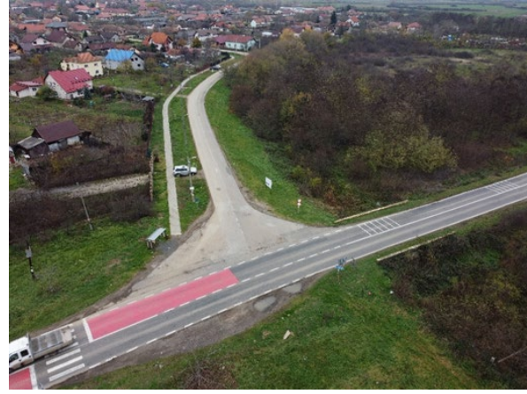
Figure 4 Intersection with county road and surface drainage channel view 2
