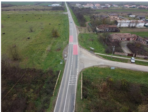
Figure 3 Intersection with county road and surface drainage channel view 1
