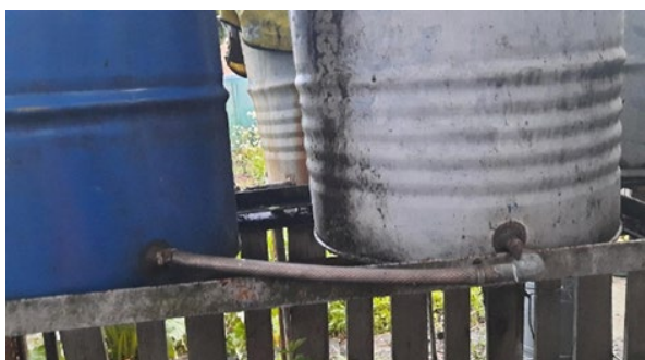
Figure 3. Example of connection of several tanks
