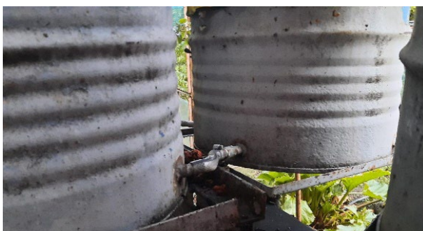
Figure 3. Example of connection of several tanks
